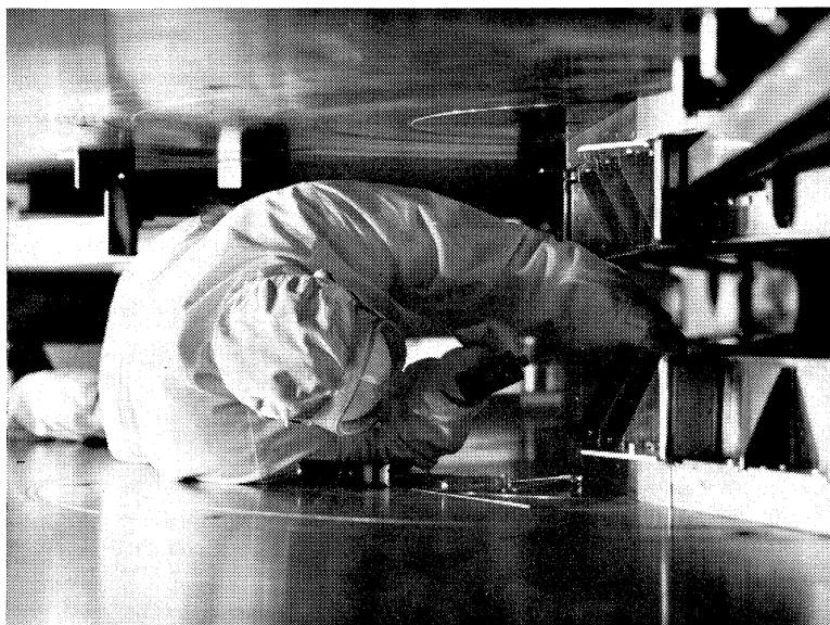
2. Because of the radioactivity inside the cyclotron vacuum tank, work there has to be carried out quickly and accurately. This is not helped by the narrowness of the gap between the two magnet poles, as this picture shows.
